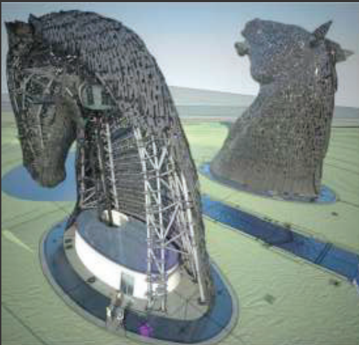
Internal Structural Design of Horse Mascots
